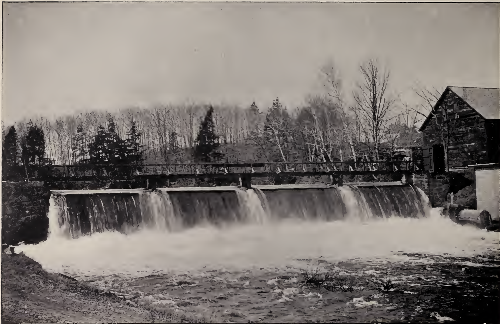
DAM NO. 5, OWNED BY THE HOLLINGSWORTH & WHITNEY CO.—FALL 16.90 FEET. See Page 35
